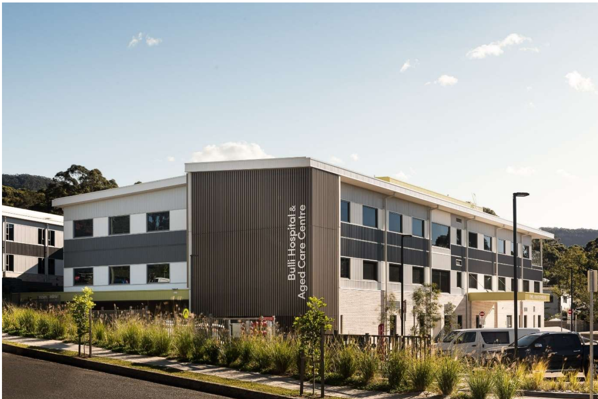
Figure 6-14: New Bulli Hospital and Aged Care Centre
