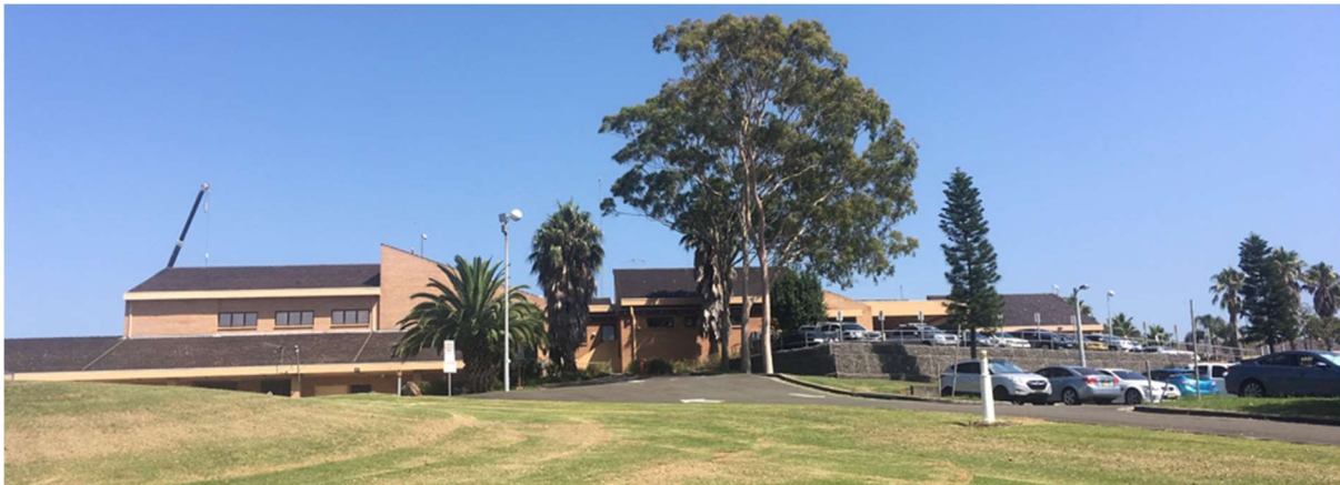
Figure 3-6: Shellharbour Public Hospital at Mt Warrigal
