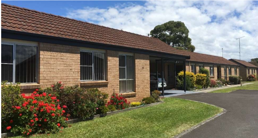
Figure 3-5: Warrigal Warilla Village units current ‘meantime use’ for 3 migrant workers
