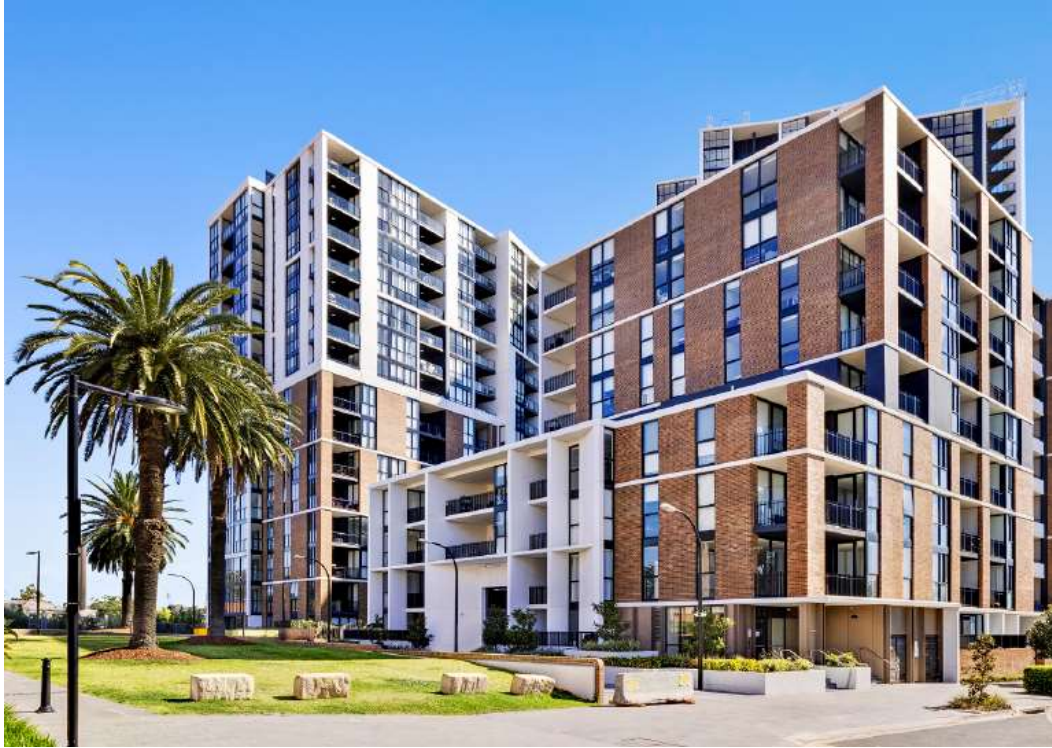
Figure 4-13: SGCH’s Key Workers Housing in Highline Development, Westmead
